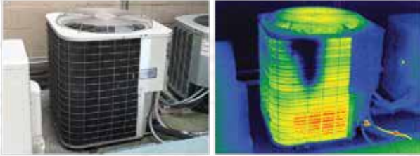
REFRIGERANT LEAKS
